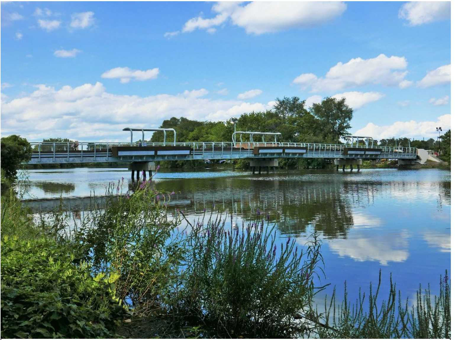
The new pedestrian footbridge connects the Teaneck and Hackensack sides of the campus across the Hackensack River. (Photo: Bill Kennedy)
